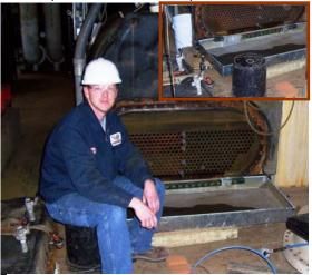
One of our Service HVAC Technicians did just that when he made a pan to collect water & debris from the chiller bundle that is being cleaned at Schlitz Park. A hose is attached to the pan to safely direct the waste away from the work area. In the past, all the water & sludge from inside the chillers would be on the floor causing a mess to clean up and creating a safety hazard. This pan, shown in the picture at left, was an easy solution to a messy problem.
